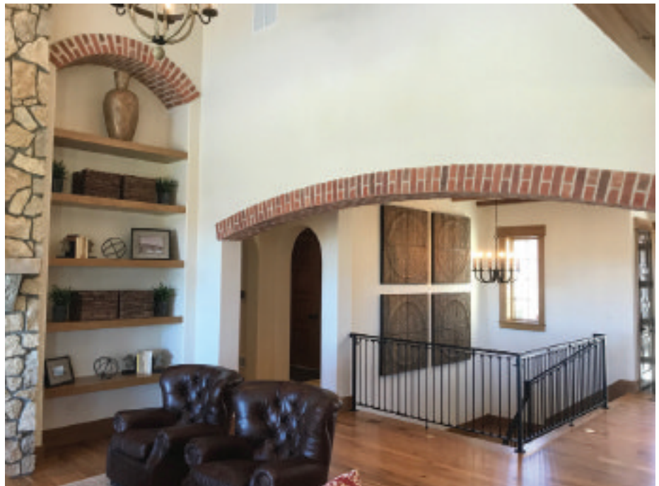
Striking, thin masonry from General Shale provides beautiful interior highlights, such as arches and accents walls and is applied in a similar fashion to tile. Photo by General Shale
